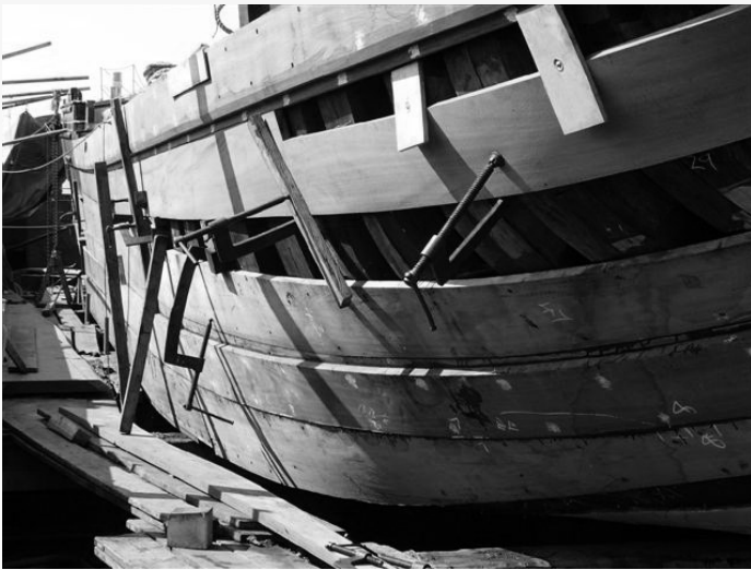
Barge being planked
