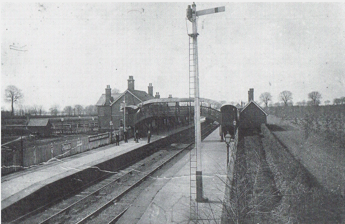
Burnham Station—The Mildmay Iron Works were built on the land to the right
